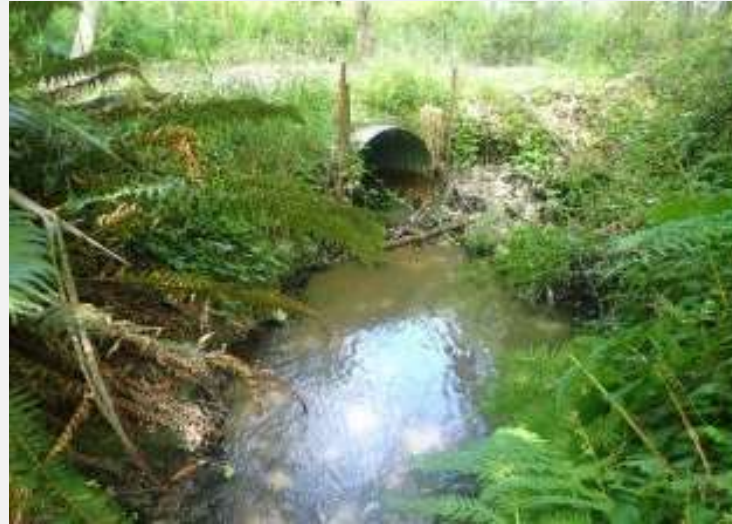
Before: Undersized culvert blocking Coho Salmon passage.
