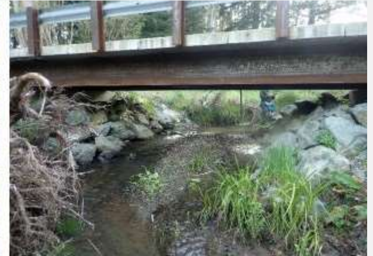
After: Thirty-foot spanning bridge with a natural channel bottom.
