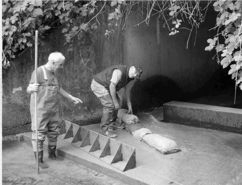
Hugh Hamilton and West Vancouver Streamkeepers installing baffling in culverts.
