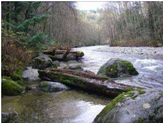
Picture showing the LWD structures placed on the main-stem portion of the Coquitlam River.
