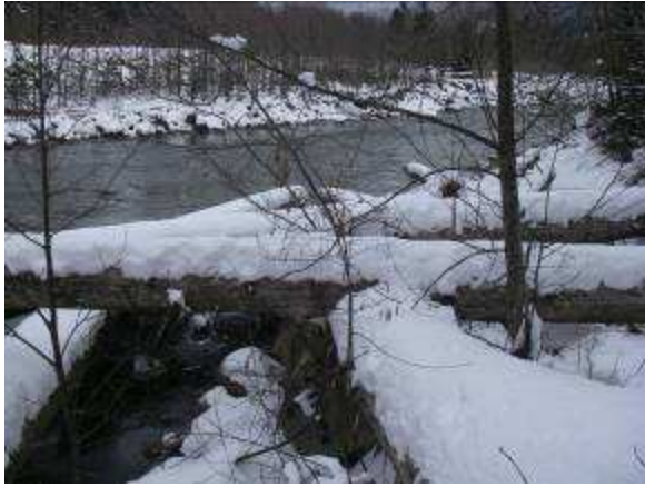
Example of a debris catcher placed on the Coquihalla River after the flood of 1995, still in place and functioning.
