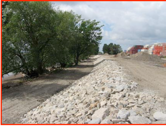
Dike bank protection construction in Richmond
