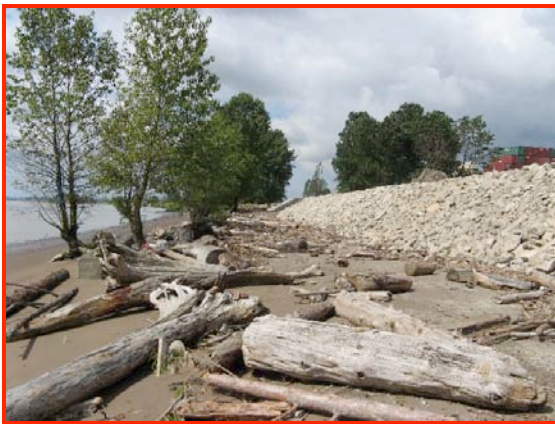
Arrangement of logs at dike toe
