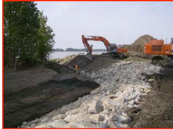
Native sediments placement on riprap
