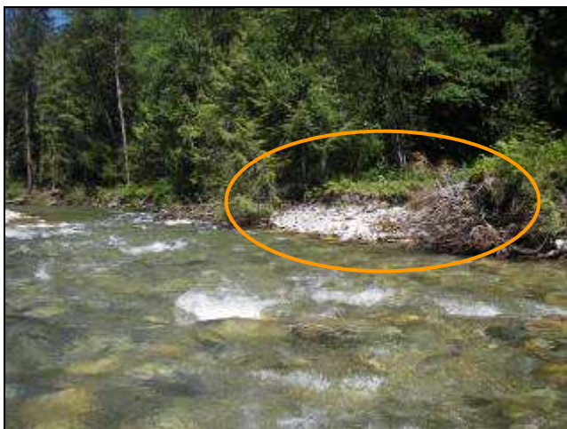
View of the downstream end of the over-flow channel where it re-enters the mainstem.
