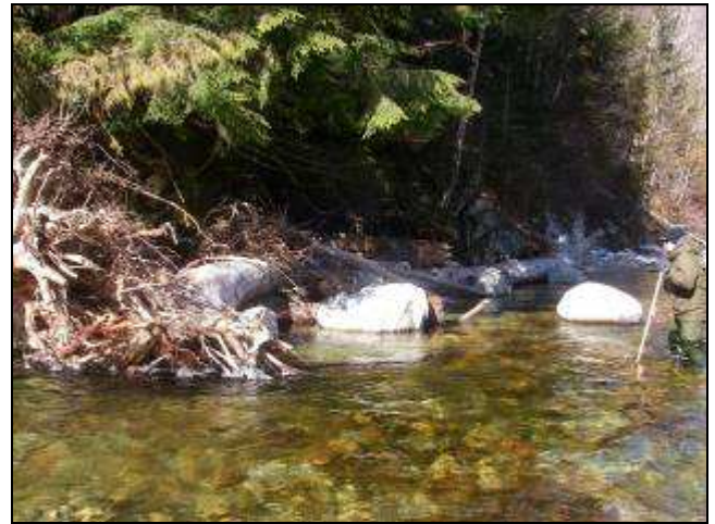
View looking downstream on a parallel wood structure which has a tree lodged against it (March, 2009).
