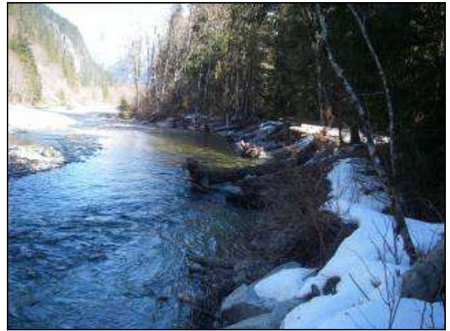
View looking downstream of the protected bank (March, 2009)
