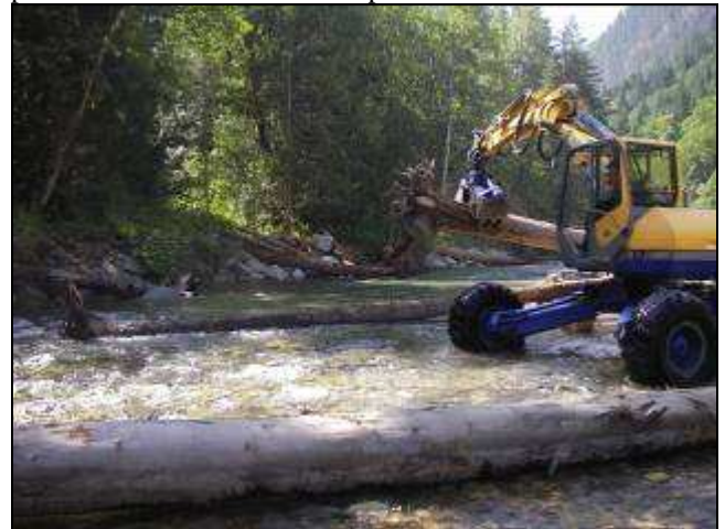
Biodegradable vegetable based lubricants are used in place of harmful petroleum based products.
