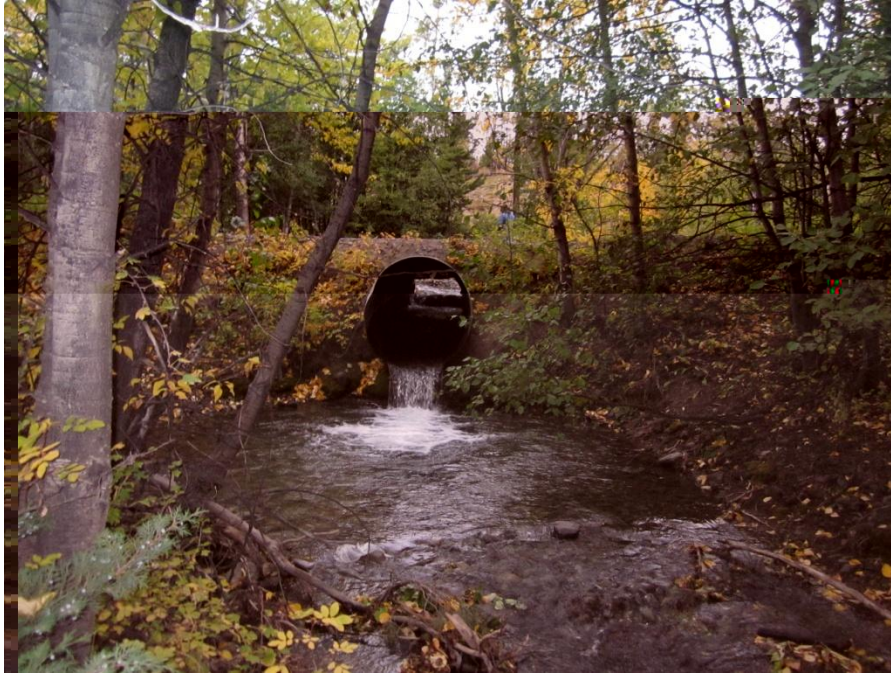
Photo 4: Drop culvert preventing upstream migration during low flows.
