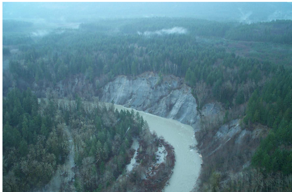
Photo 4. Aerial upstream view of the Stoltz slide that extends for 600 m along the left bank for the mainstem Cowichan River. Remedial works undertaken in 2006 and 2007 have successfully reduced erosion and sedimentation (Sheng and Bonnell 2010).
