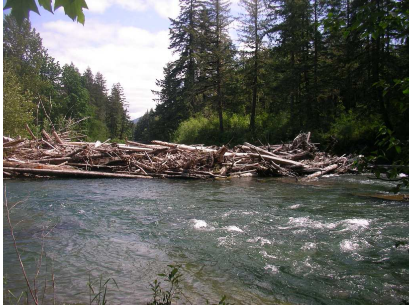
Photo 5. Downstream view of the entrance to Skutz Falls and the fishway illustrating the large woody debris accumulation that requires annual maintenance to facilitate upstream migration of spawners (Sheng and Bonnell 2010).
