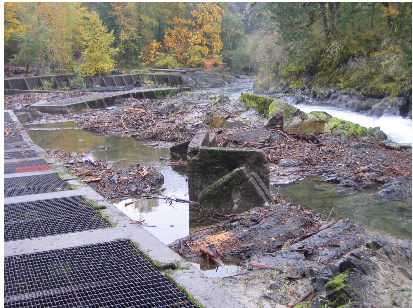
Photo 1. Downstream view of Skutz Falls illustrating the vertical slot fishway constructed in 1956 (Sheng and Bonnell 2010).
