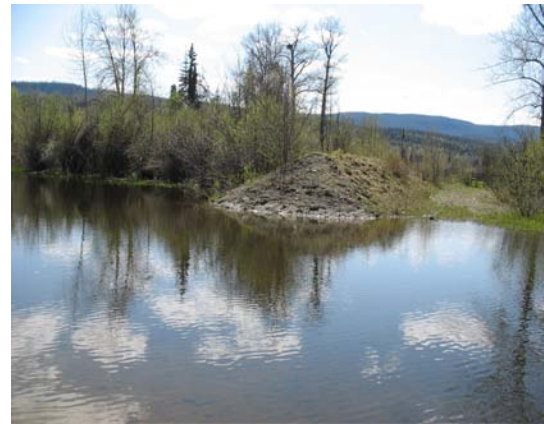
Figure 4. South toe of dyke breach
