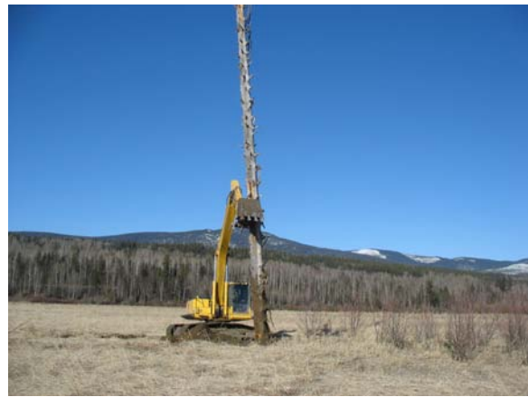
Figure 15. Planting of new snag
