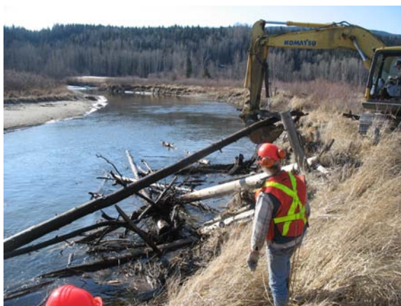
Figure 12 and 13. Removing debris catchers along the main stem of the Horsefly
