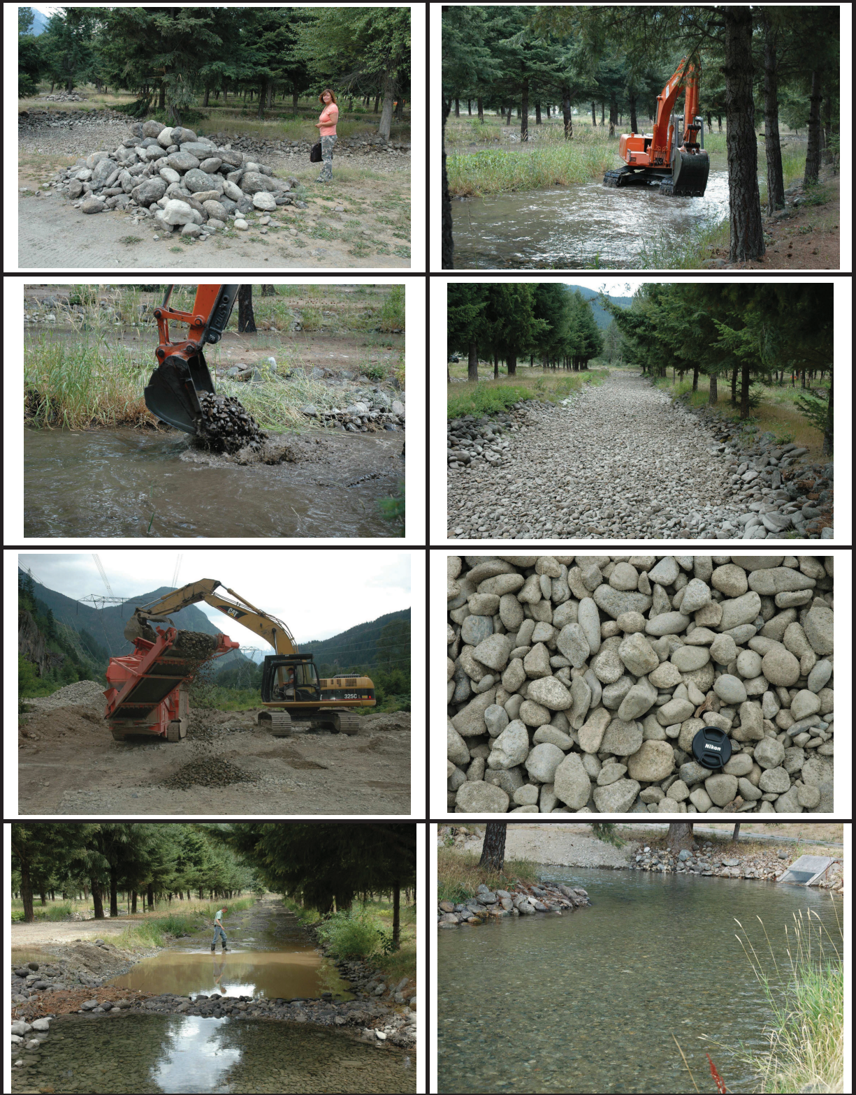
Methods utilized during the Gates Creek spawning channel gravel replacement project.
