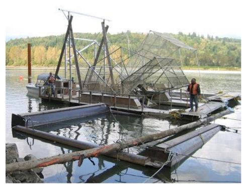
Figure 18. Photo of the Crescent site showing the position of the floating shoreline abutment, fishwheels, and barrier net (attached to the orange float in the background), 8 October 2008.
