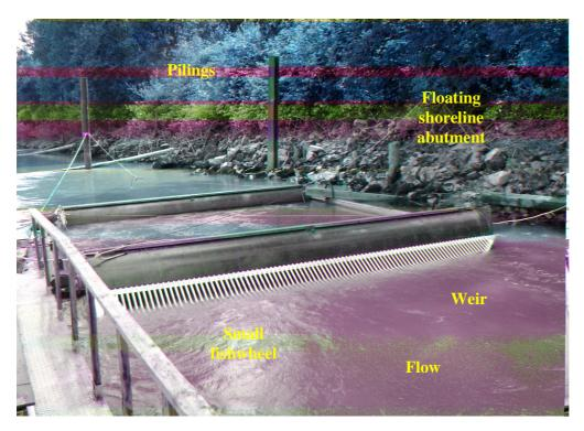
Figure 5. Floating shoreline abutment and weir at the Crescent fishwheel site, 7 July 2008.
