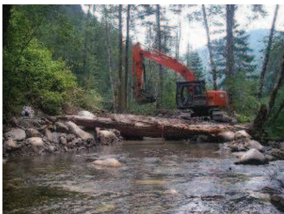
EXCAVATOR MAKING ADJUSTMENTS TO INTAKE STRUCTURE TO PROVIDE GREATER FLOWS
