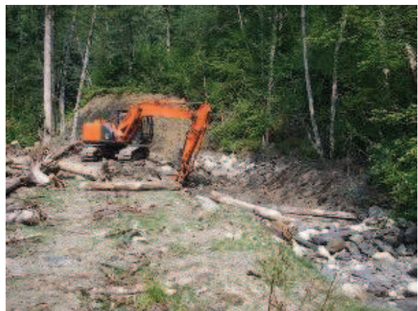
BUILDING RIFFLE HABITATS AND ARMOURING BANKS IN THE UPPER PORTION OF THE CHANNEL
