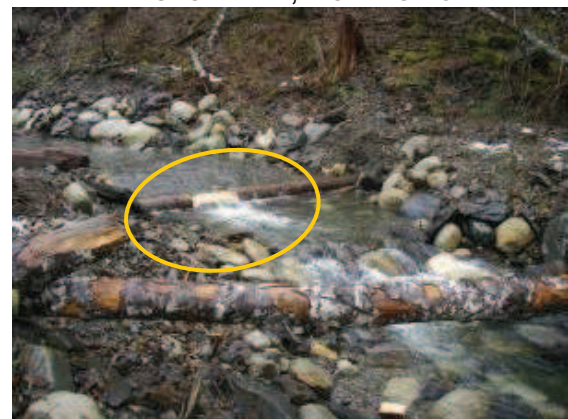
LOG DROP STRUCTURE REFINED BY NOTCHING THE LOG TO DIRECT A FLOW AND IMPROVE FISH PASSAGE
