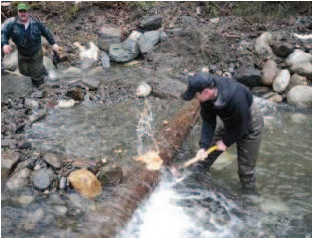
Notching out a log drop structure to direct the flow (Fly BC; Photo posted by Tex)
