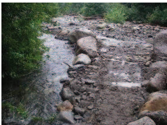
OVERFLOW OUTLET WAS DESIGNED TO ALLOW SILT-LADEN WATER (DURING HIGH FLOWS) TO EXIT THE CHANNEL AND LIMIT SEDIMENT DEPOSITED INTO THE LOWER CHANNEL
