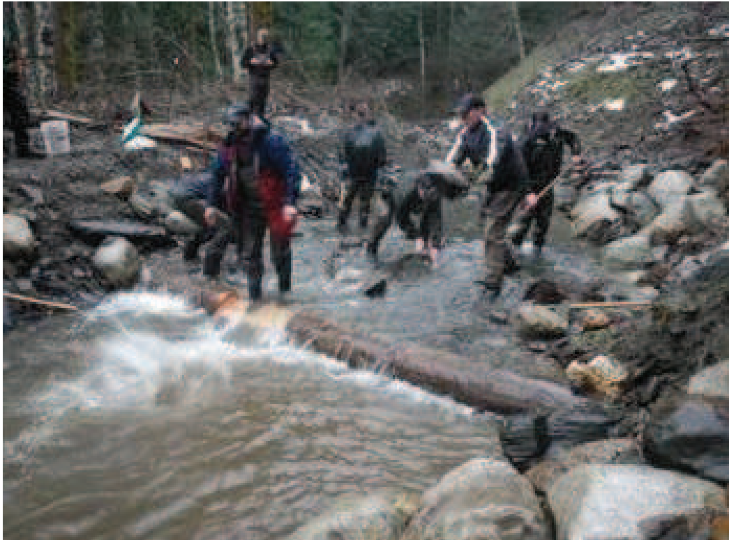
Finished product at the drop structure (Fly BC; Photo posted by Tex)
