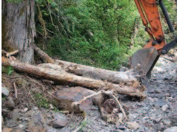
BUILDING ONE OF THE TRIANGULATED LWD STRUCTURES
