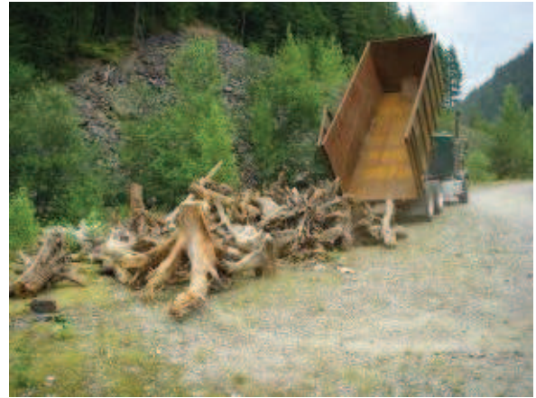
LARGE BIN TRUCK OFF-LOADING LOGS AND STUMPS TO BE SET FOR AIRLIFT INTO THE CHANNEL COMPLEX
