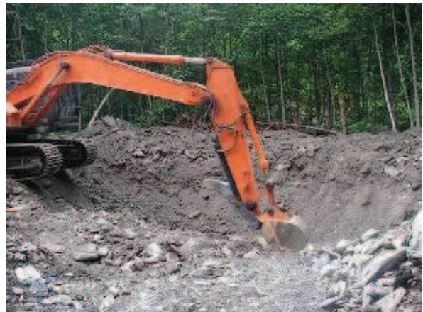
EXCAVATING A LARGE POND IN THE UPPER PORTION OF THE SIDE CHANNEL
