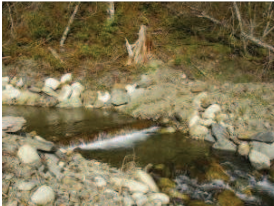
LOG DROP STRUCTRE POSITIONED TO AID IN POOL DEVELOPMENT BELOW THE STRUCTURE
