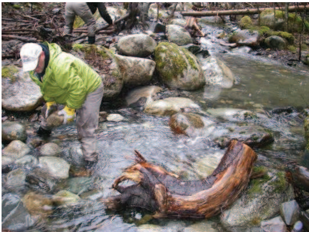
Creating a small riffle to backwater and improve access at the riffle immediately upstream
