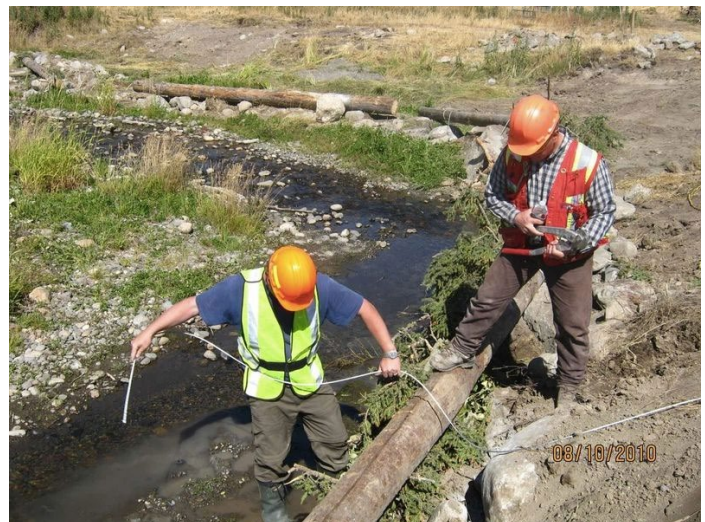
Live bank protection (Photo credit: Wayne Salewski)
