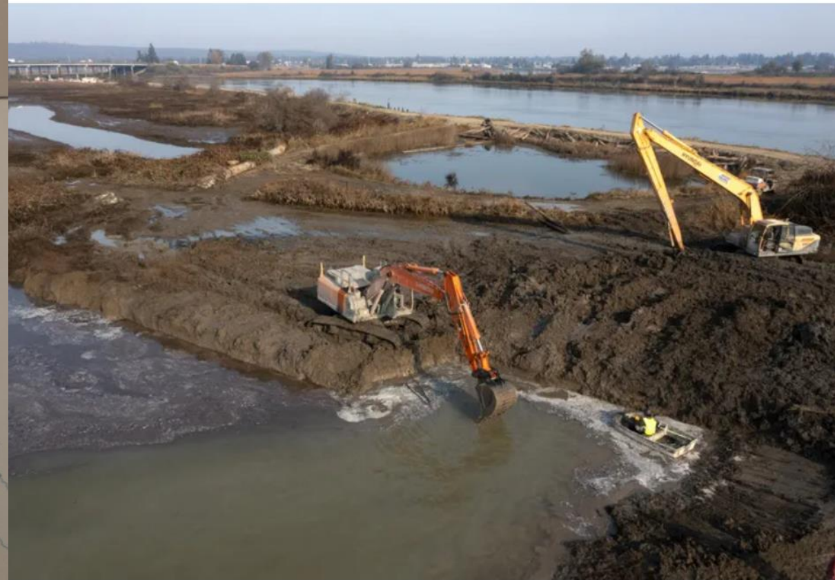
1 of 4 | Excavators work on breaching the final dike in the Blue Heron Slough restoration project in Everett on Oct. 3. A levee separates Steamboat Slough, on the right, with farmland that's being dug out at low tide. (Karen Ducey / The Seattle Times)
