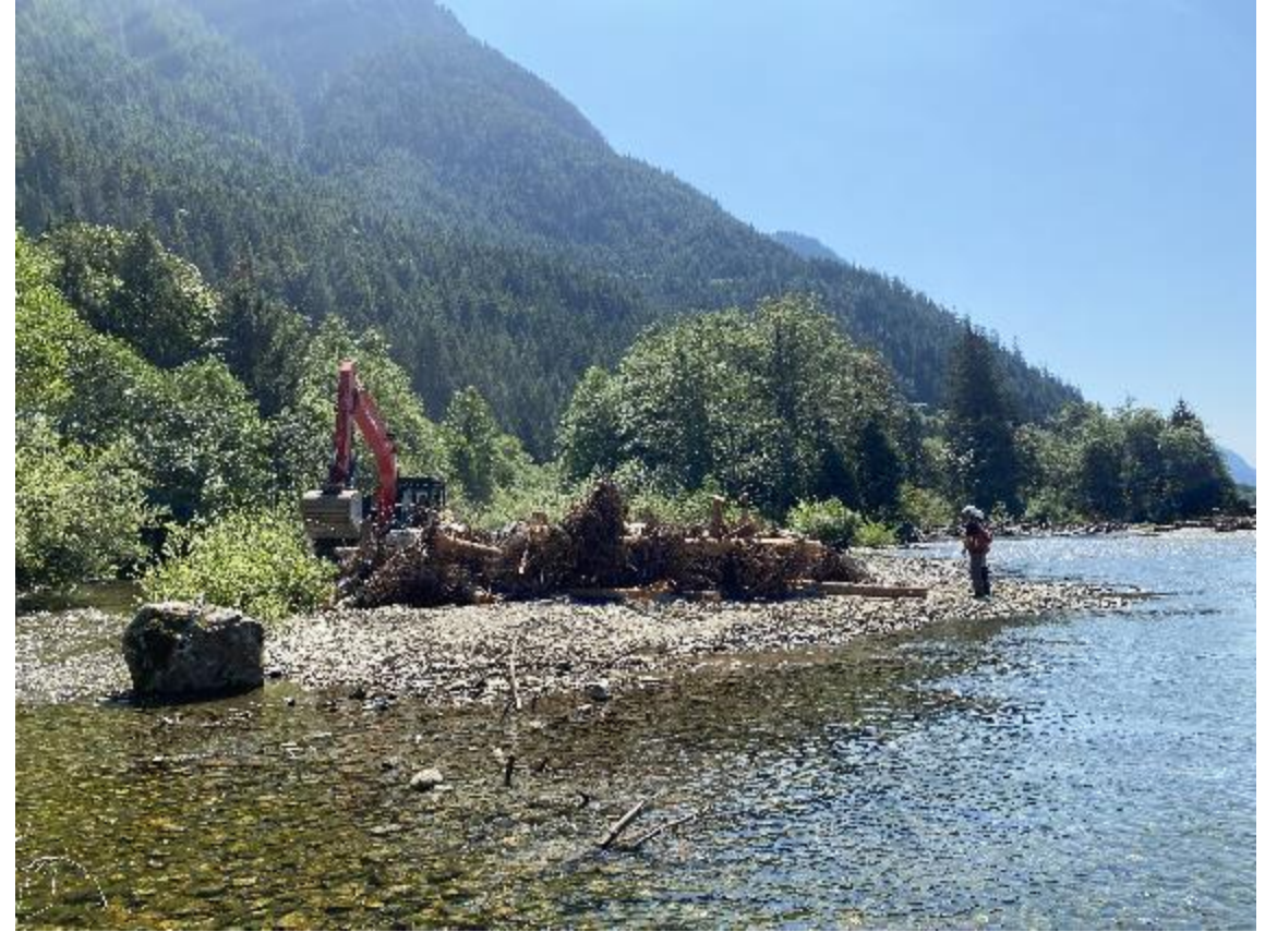
View downstream / south
