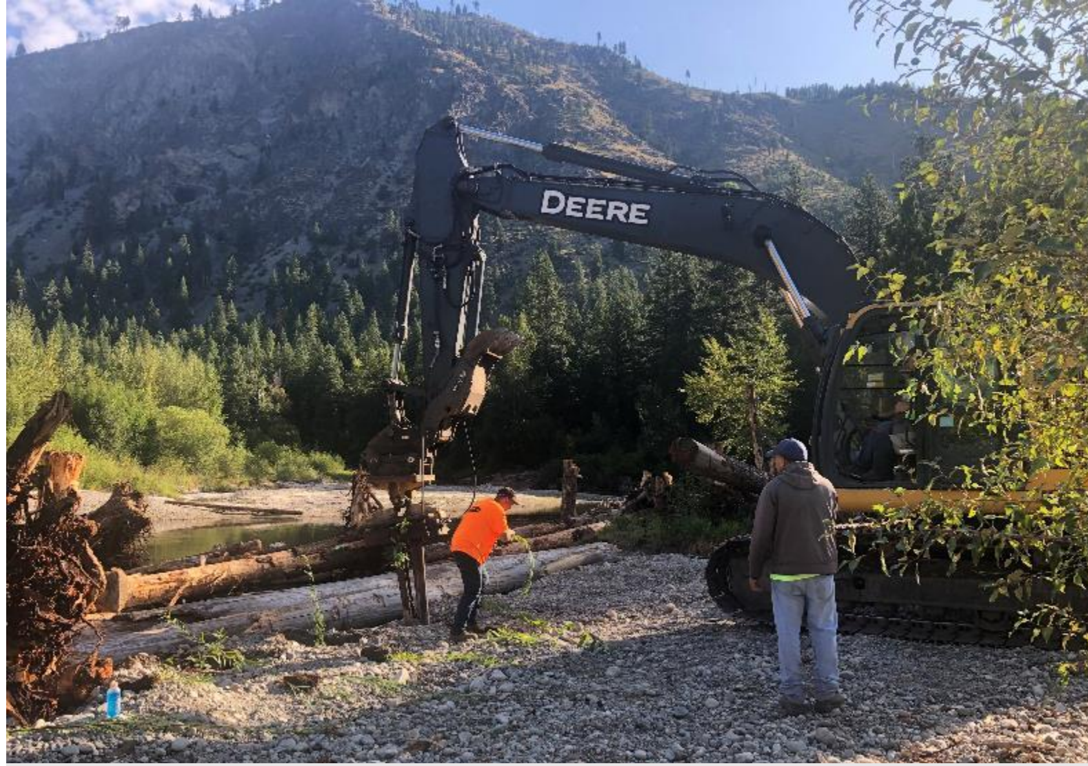
RM 21 Mechanical Planting in gravel bars with Stinger at former levee
