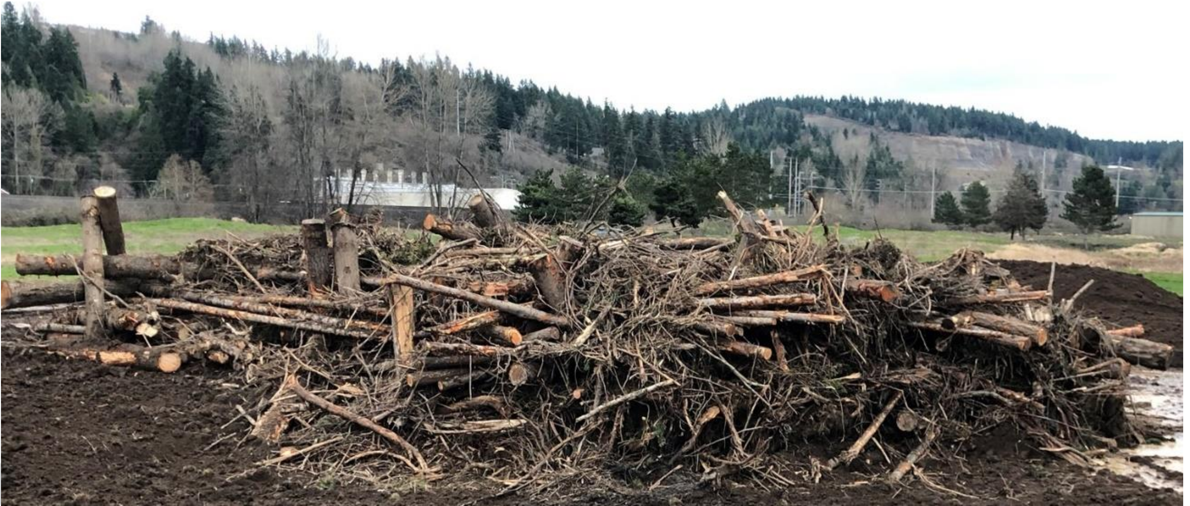
Lower White prototype structure City of Sumner, WA
