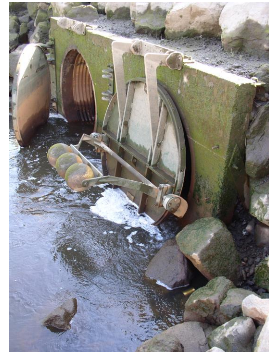
Top-hinged TG with Mitigator Device
