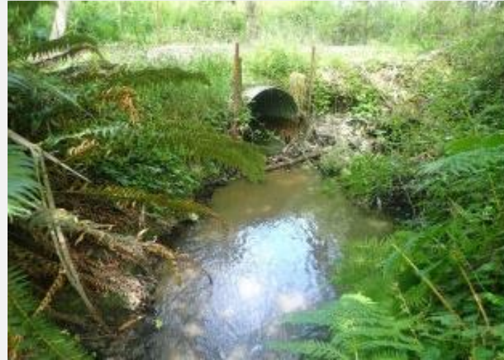
Before: Undersized culvert blocking Coho Salmon passage.
