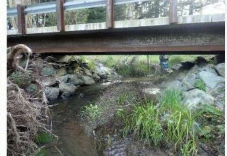
After: Thirty-foot spanning bridge with a natural channel bottom.
