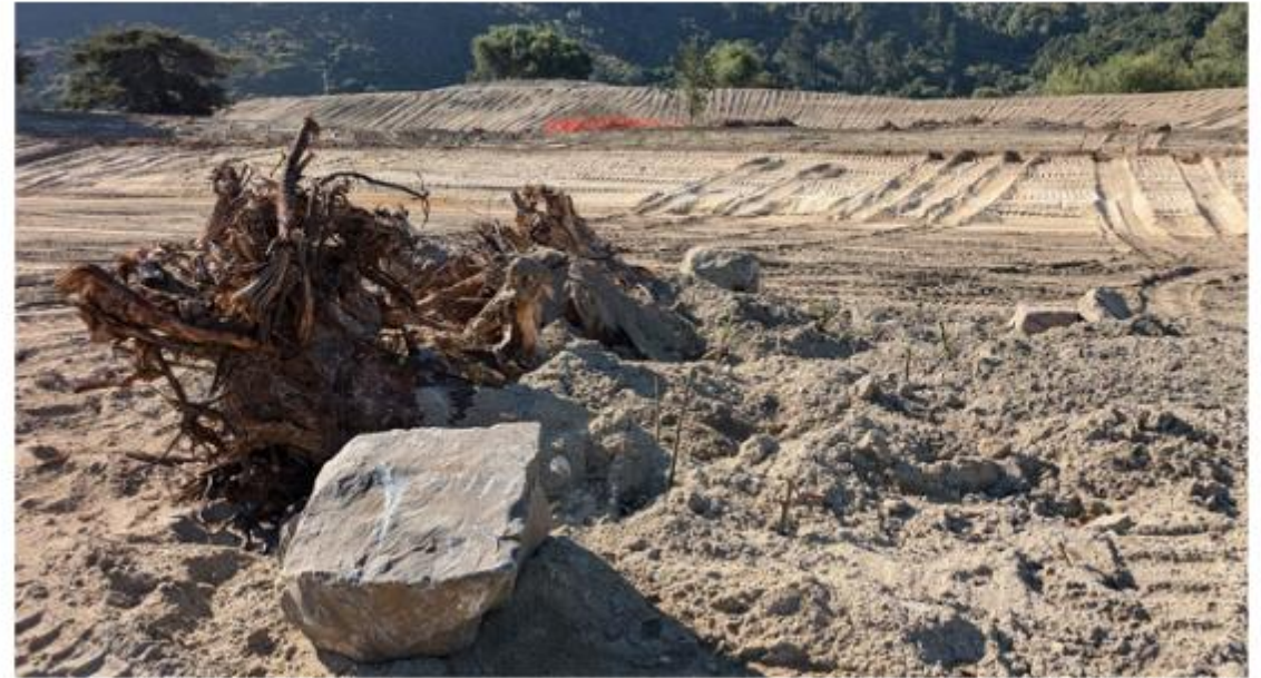
Figure 10: Wood habitat structure. The logs are buried under the floodplain in trenches with boulder ballast to reach stability.
