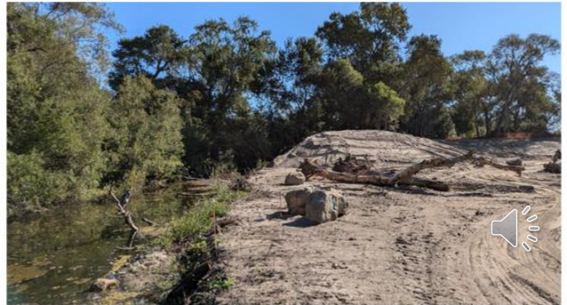
Figure 11: Downstream floodplain connection near Bridge 4 on 8/28/2025, looking north. Large wood is staged for wood feature #1 to be installed after the Carmel River is dry. Note great blue heron on snag in the river channel, unperturbed by construction.
