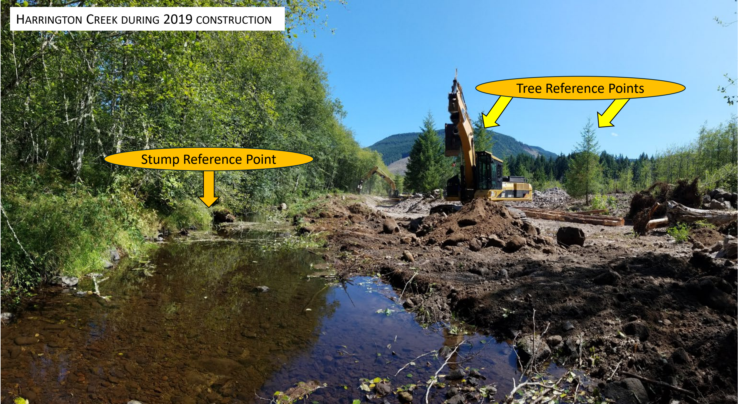
WE TOOK ABOUT 3 FEET OFF THE ADJACENT FLOODPLAIN SURFACE. NO DEWATERING OR REMOVING FISH FROM THE CHANNEL WAS REQUIRED. WE LEFT ISLANDS WHERE 20-30' TALL DOUGLAS FIR TREES WERE ALREADY ESTABLISHED (SEE YELLOW ARROWS).
