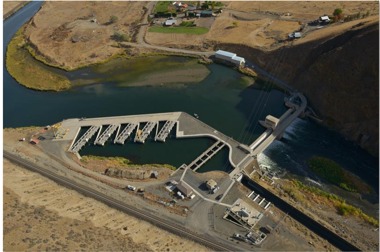
Roza Diversion Dam and fish screen facility. (Photo by Kirsten Strough | Reclamation)
